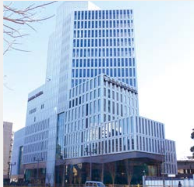
A view of Bldg. 6 from Kojimachi-Odori
